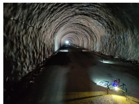
Tunnel tests configuration (EURECAT)
